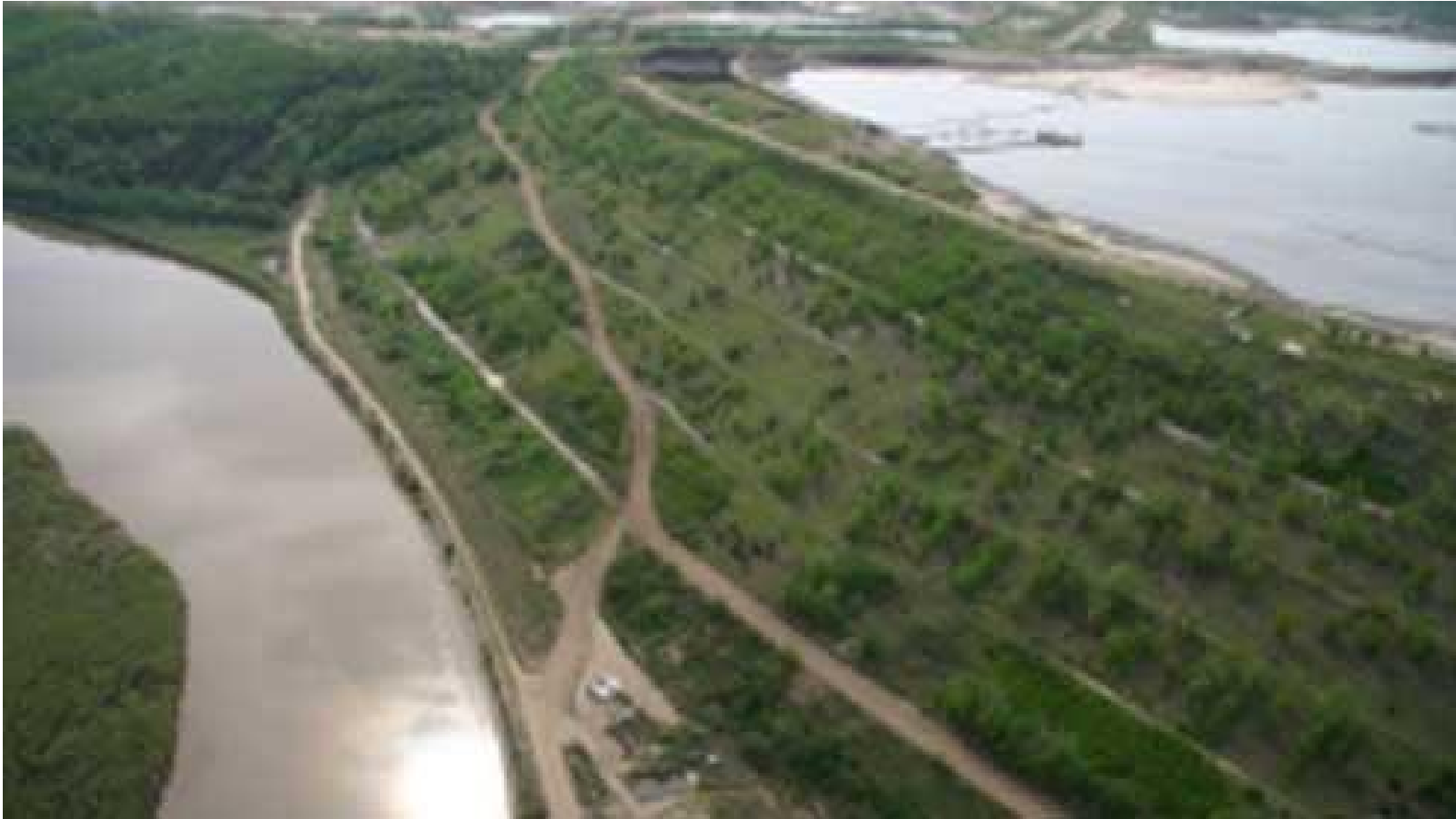
Suncor's Tar Island Tailings Dam
